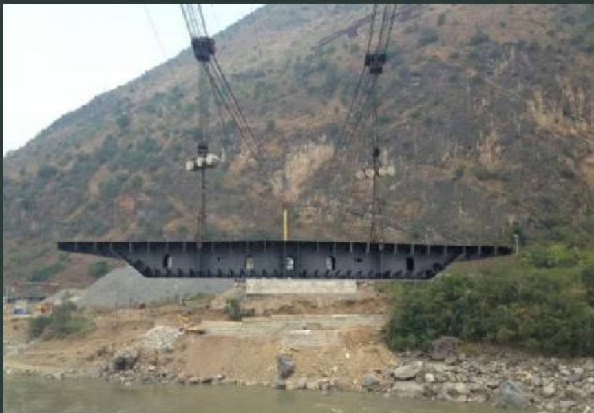
缆索吊机拼装架设
