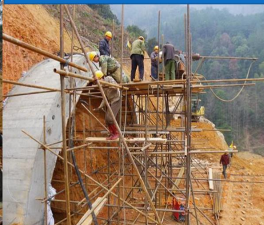
6.套拱拆模后施钻管棚孔
