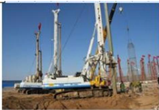
旋挖法施工
